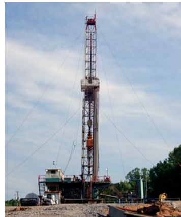
5/11, Middlesboro, SE KY, drilling for gas below Pine Mtn. thrust
